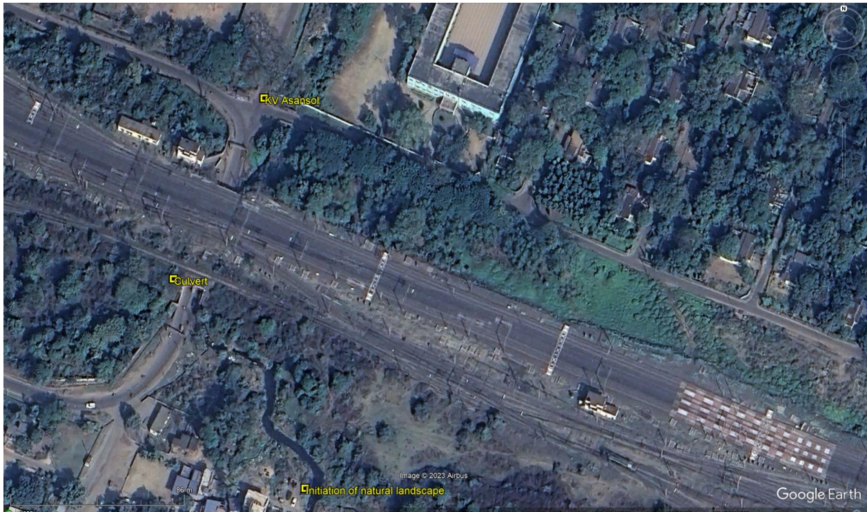
Figure 4: The survey continued where the river meandered across the natural landscape, leading to the culvert connecting old and new Asansol, and ending adjacent to the boundary of Kendriya Vidyalaya, Asansol.
